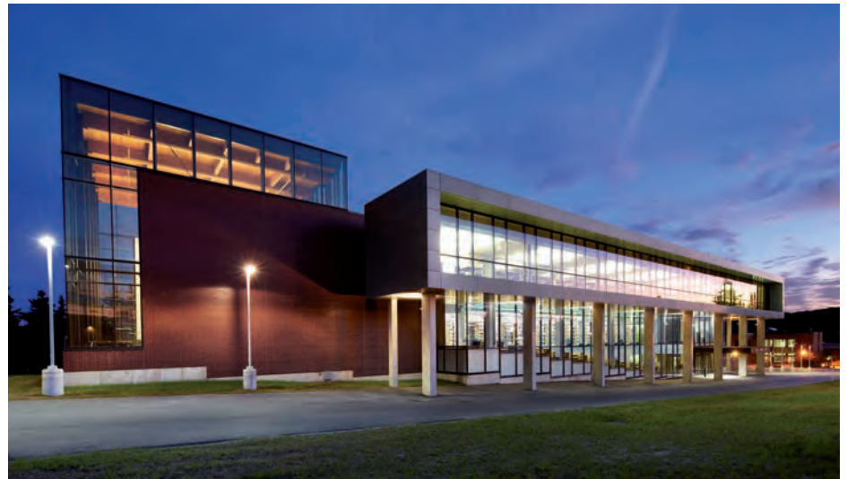
Mass timber expression, panel cladding and glazed walls complement brick
