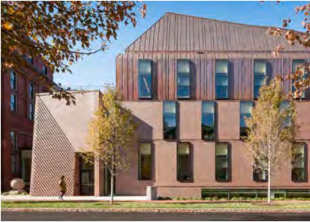
Modernization of brick expression with fabrication and high-performance glazing
