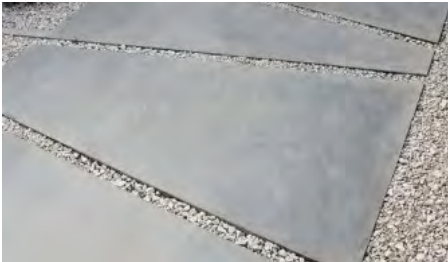
Pre-cast concrete pavers and cast-in-place slabs (above)
