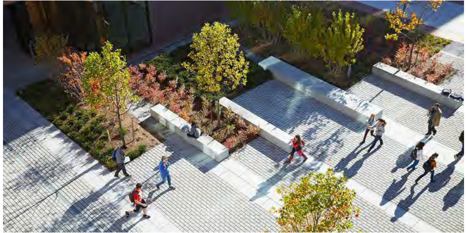
Hardscape Plaza at University of Connecticut New Social Sciences by Stimson Studio (Photography: Charles Mayer)
