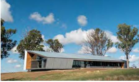
Warm-but-sleek form and materials and low-impact foundations at field buildings
